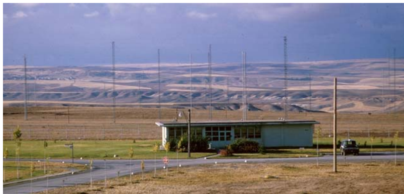
The PMO and part of the huge antenna field at Det 27
